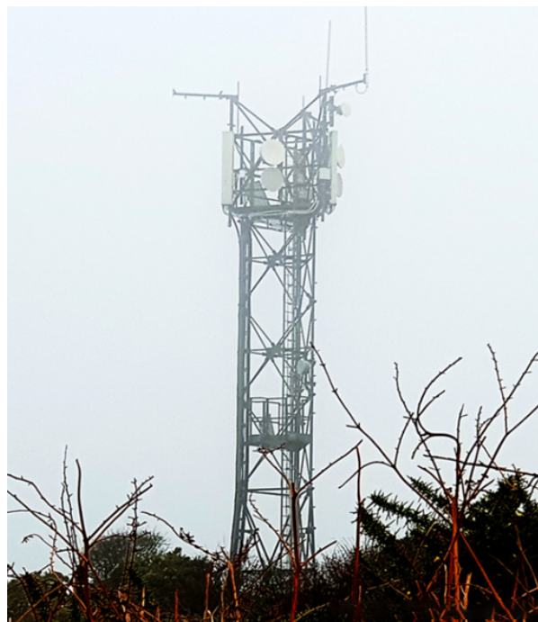
"Mast in the Mist"! Mast-mounted, multi-protocol BSNs including MPT-1327
